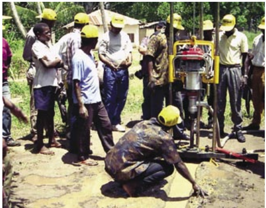
A reduced-diameter drill rig in operation.
