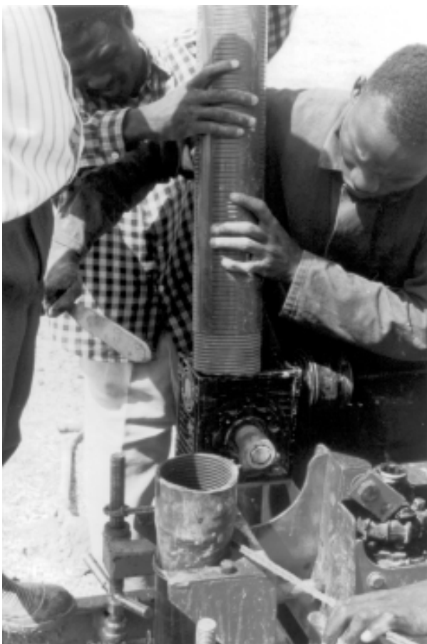
Figure 7.4 Threading uPVC casing held securely on rope wraps
