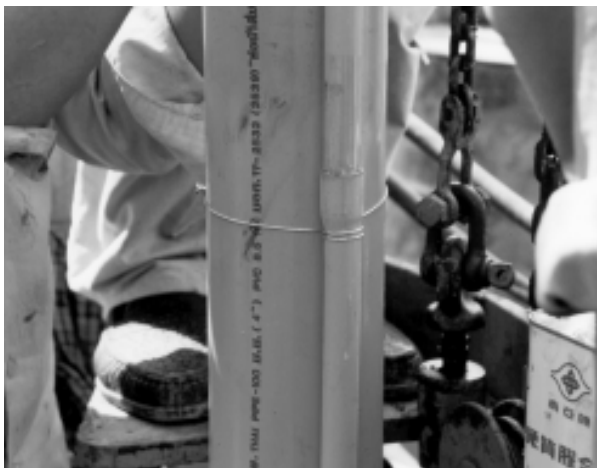
Figure 7.17 Use of small diameter pipe as centralisers
