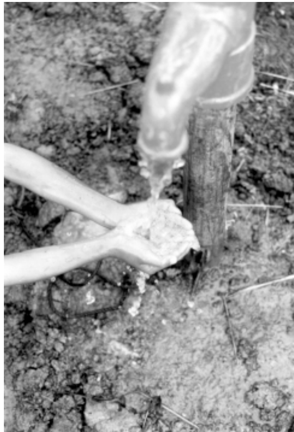
Figure 9.3 Borehole properly developed and sealed ready for handover to user
