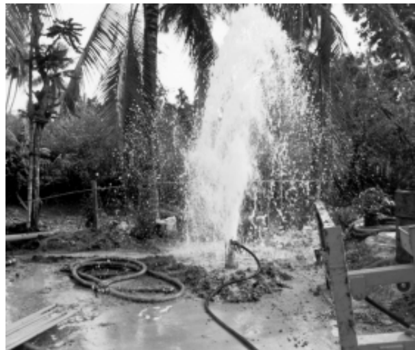
Figure 7.12 Final stages of developing with compressed air
