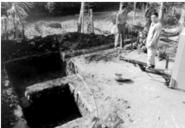
Figure 2.5 Well proportioned mud pits ready for filling
