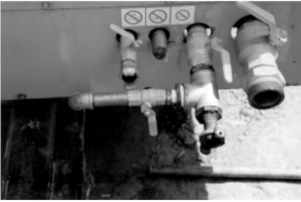
Figure 7.11 Air development manifold – Allowing discharge to atmosphere
