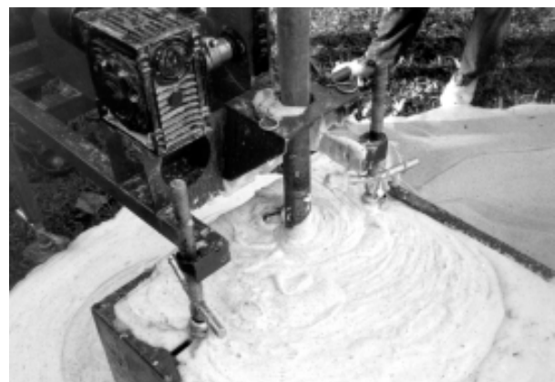
Figure 4.1 Drilling with stable foam
