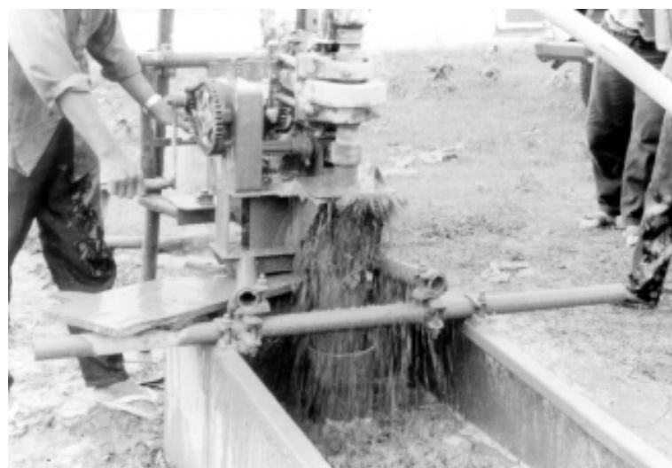
Figure 3.2 Drilling with compressed air – having "struck" water
