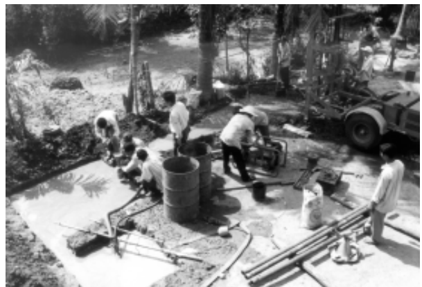
Figure 2.6 Functioning mud pits – slow moving flow for good settlement
