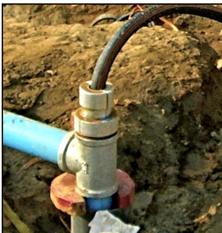
Tee piece with locker clamps & hose
